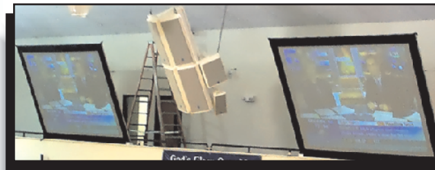
Integrated Audio Video System being installed in Sports / Worship Facility
